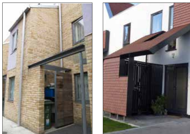
Fig 5.27: Simple porches designed to incorporate bins provide convenient storage and keep bins out of sight.
